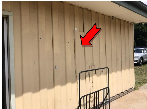
Photo 4. Exterior, croquet club, wall cladding – asbestos-containing fibre cement sheeting.
