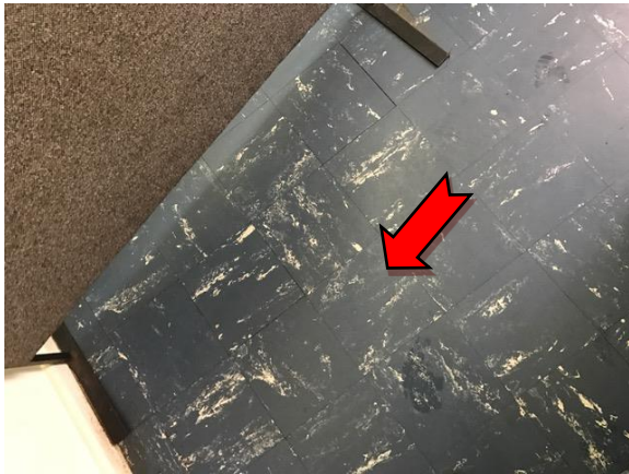
Photo 3. Interior, ground level, family room, blue floor covering – asbestos-containing vinyl floor tile.
