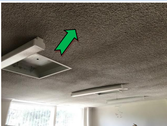
Photo 5. Interior, ground level, office and service area, ceiling – non asbestos-containing vermiculite.
